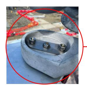
Red phase connection as found, nuts were found hand tight and spring washer not installed on centre fixing.
