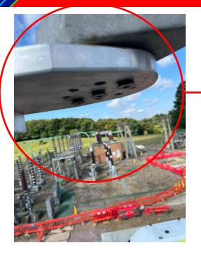
Countersunk fixings installed on flat connection, this palm joint is believed to be installed upside down.
