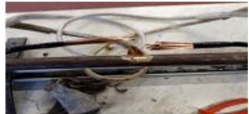
Picture 2 : Neutrals lifted and underlying conductor tested
