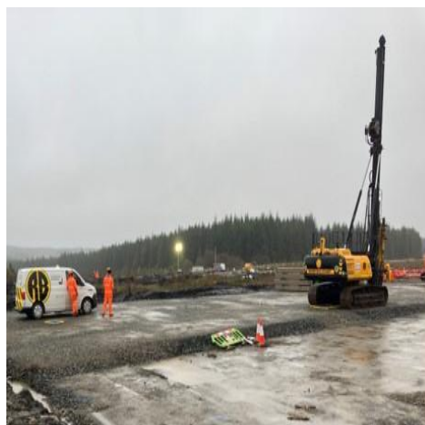
Requirement to hand-dig trial holes in advance of piling works
