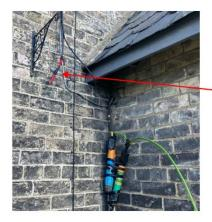
Polarity of surface wiring not identified or marked.
