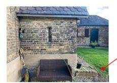
Earth Stake installed incorrectly.
