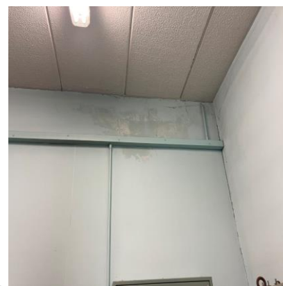
Water Damaged RAAC
