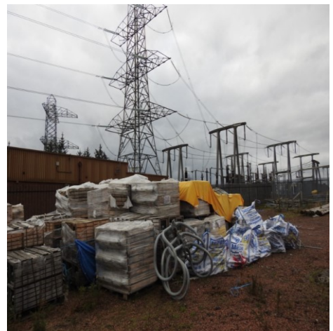
Materials stored with loose coverings in a substation
