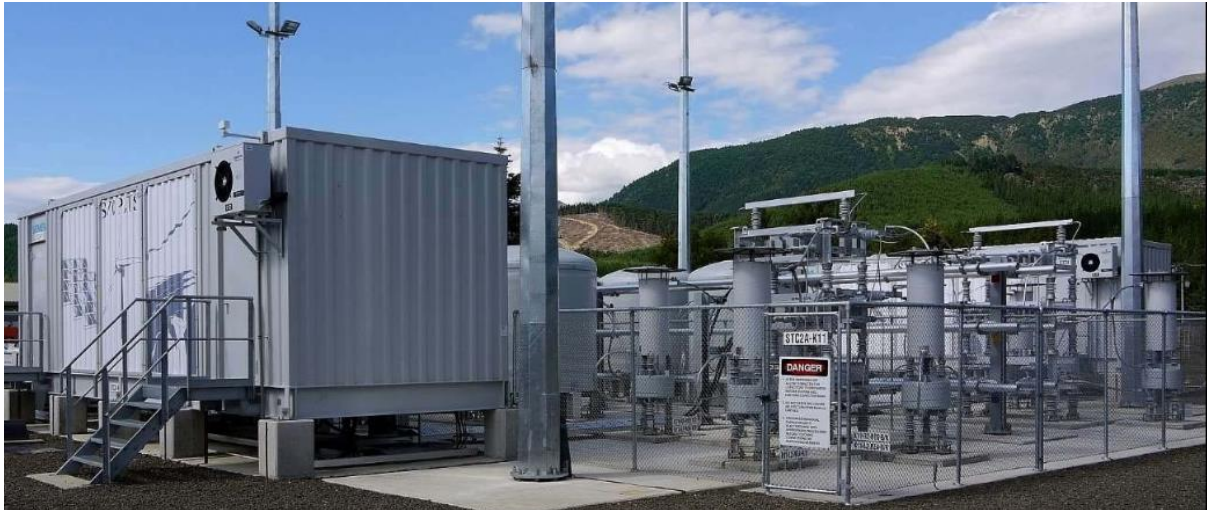
Figure 15: 40 Mvar converter container
