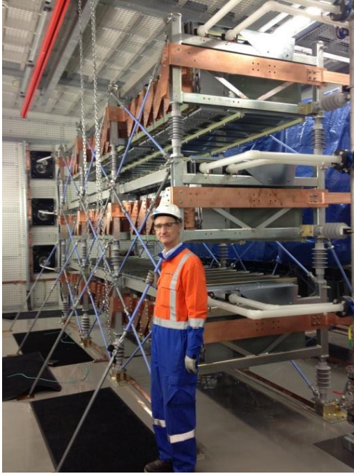
Figure 6: Left half converter stack at Haywards
