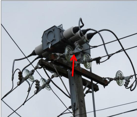
Fig. 1 Arcing caused by a gap
