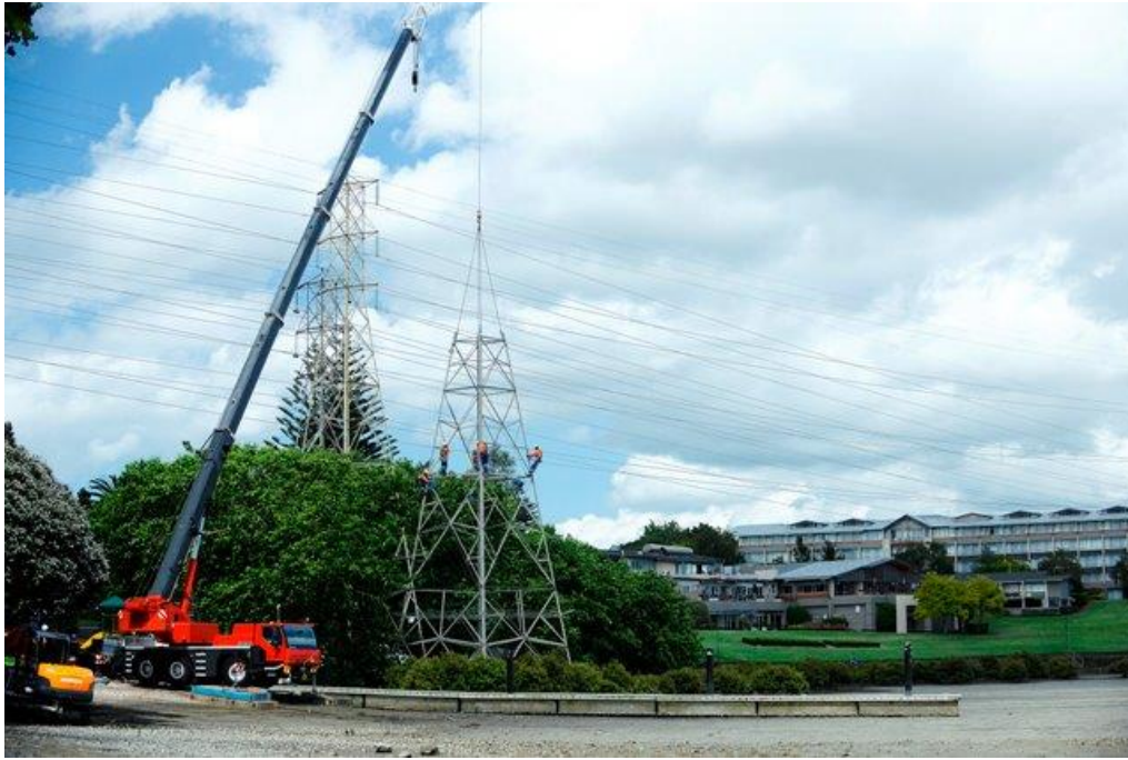
Figure 9: Tower dismantling (PAK-PEN)
