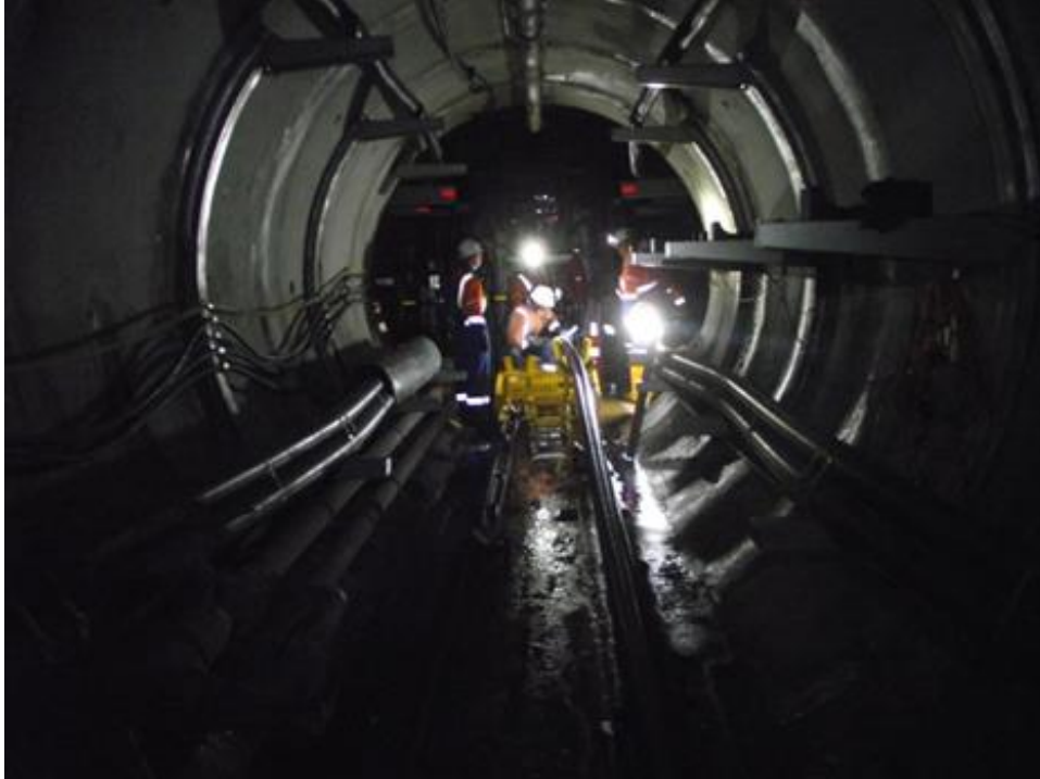
Figure 8: Installing cables in the HOB-PEN tunnel
