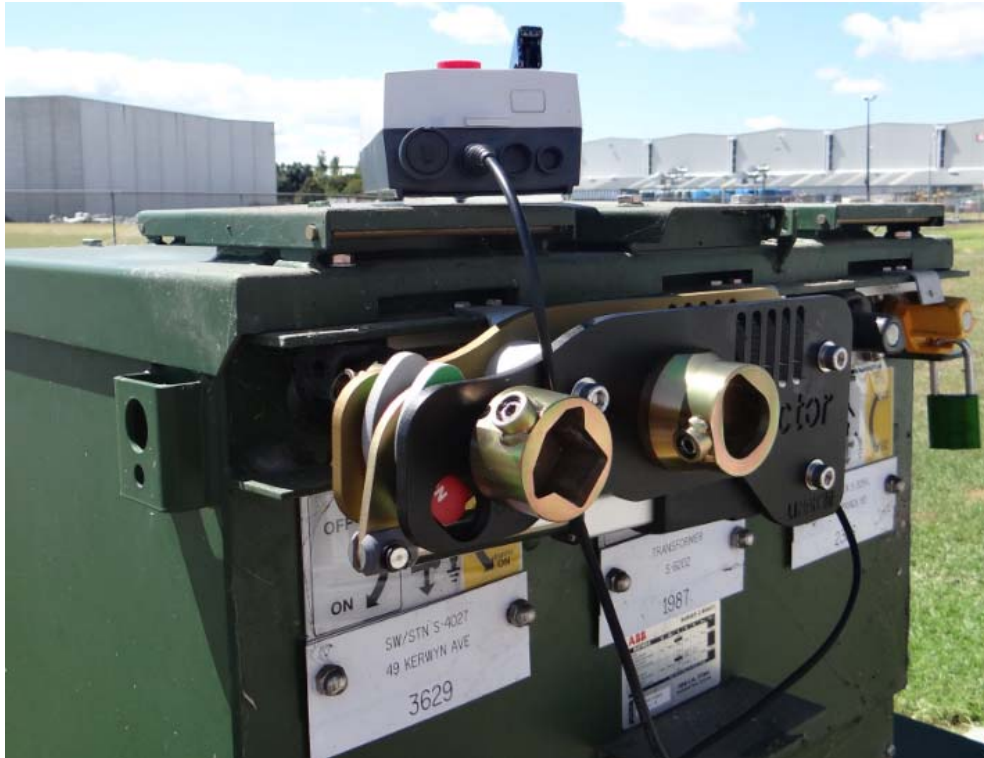
Figure 7 Portable Actuator plugged in to the Control and Battery Unit
