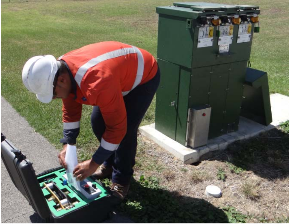
Figure 4 Site Preparation for Application of Portable Actuator
