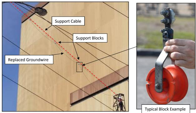
The stringing methodology was worked through in detail to confirm procedures and parameters for pull-out of the CSS, reconductoring with the OPGW and removal of the CSS. The general methodology agreed for installation of the OPGW using the CSS is:
