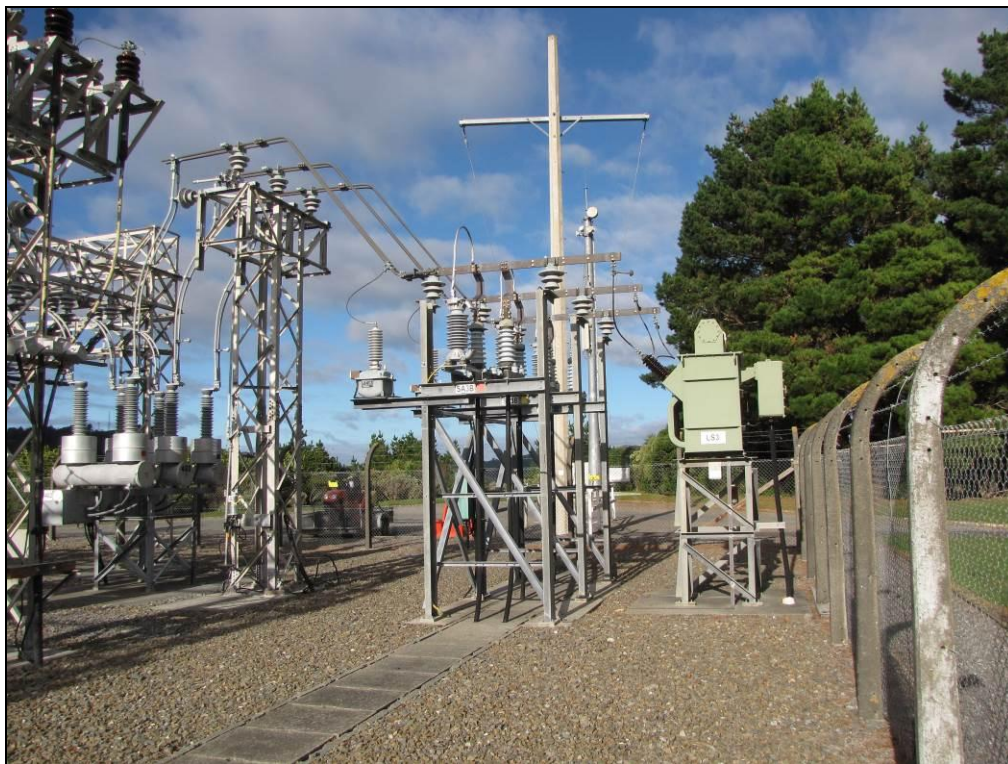
Figure 5: T3 33 kV Incomer Cable Termination Stand (before)
