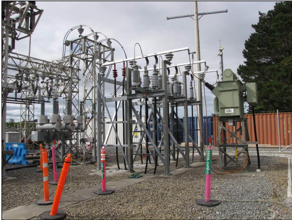
Figure 6: T3 33 kV Incomer Cable Termination Stand (after) – Extended with Additional XLPE Cables
