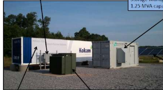
Battery container 750 kWh/250 kW Lithium Polymer battery Includes Batt. Management System
