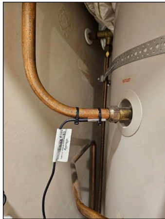
Shelly temperature probe installed on outlet pipe in house 10
