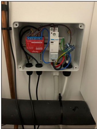
Shelly device installation in house 8
