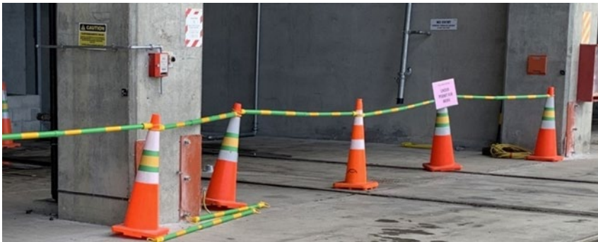
Figure: 3 Example of permit area boundary marker
