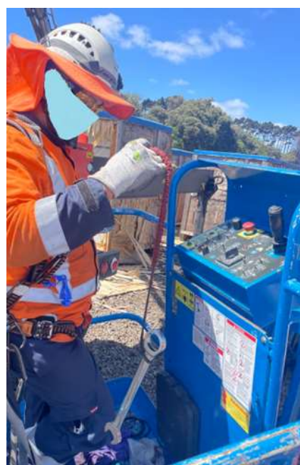
Worker on MEWP using tool tether
