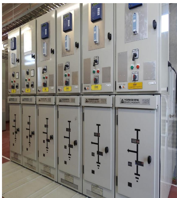
Figure 2: YSF6 indoor, metal enclosed switchboard at Tatua Substation
