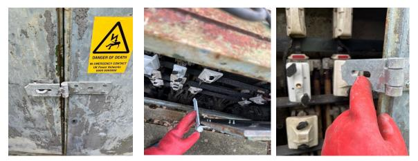
Please ensure that whenever access is made into this type of equipment, secured with a hasp and staple arrangement that the hasp is folded back on the outside of the door and the door with the staple is always closed first thus preventing the hasp from folding inwards towards the live lv bars / contacts.
