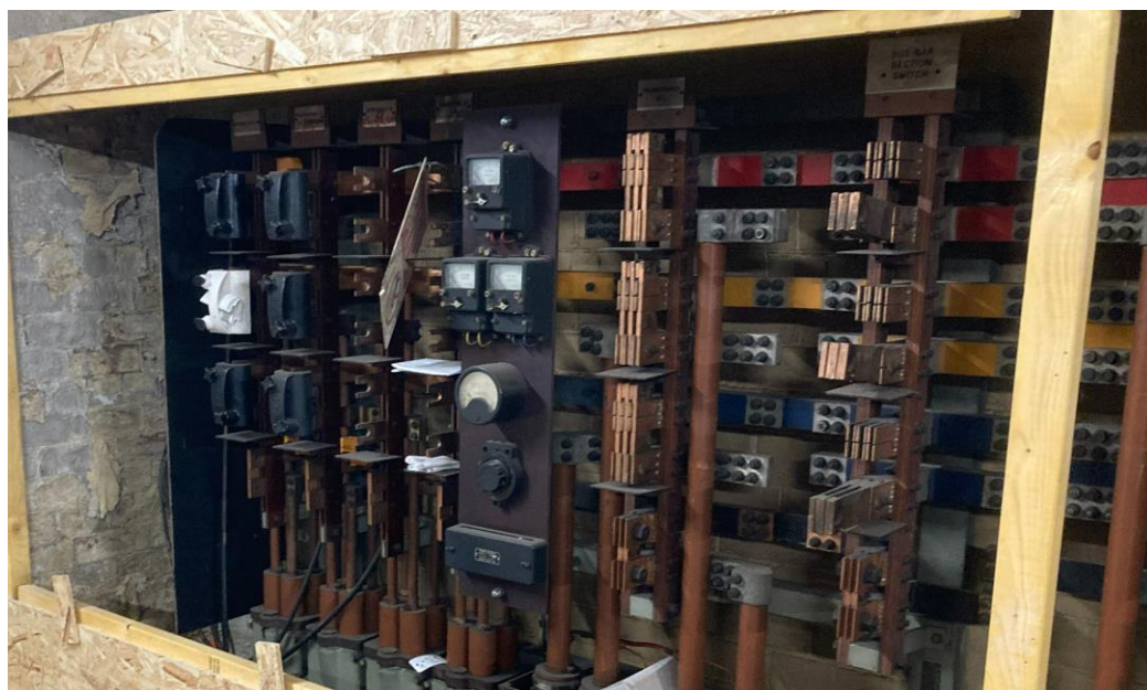
Example of open pattern LV board with hinged links
