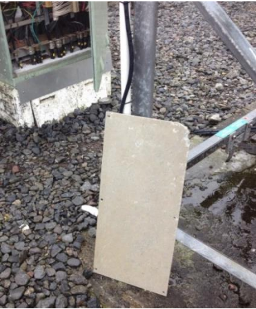
Circuit boards, OJJB panels
