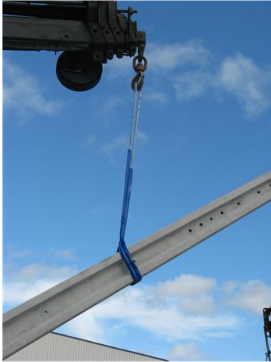
Erecting with polyester or composite material sling strop
