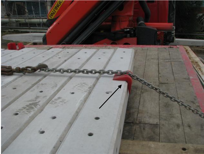
Corner protectors under chains
