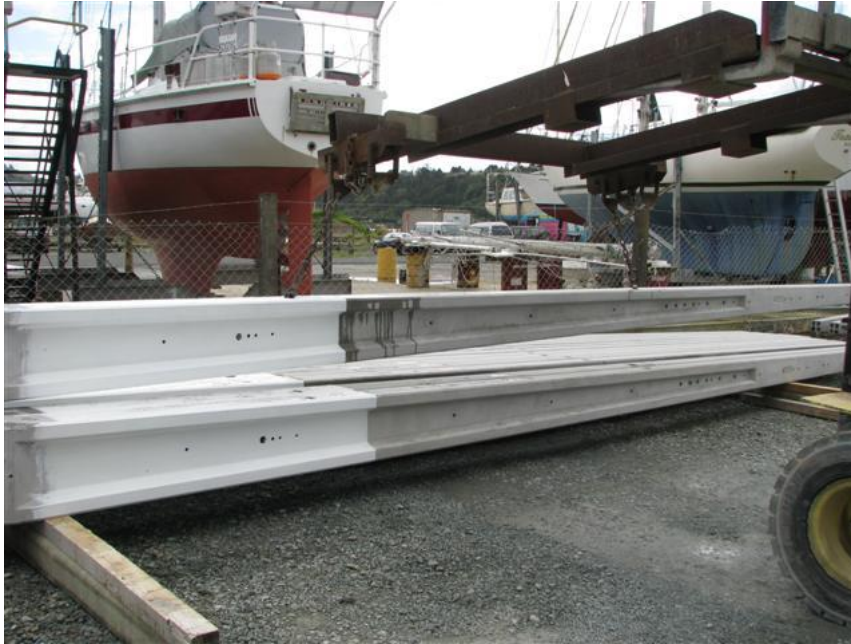
Lifting with forklift and Swift Lifts
