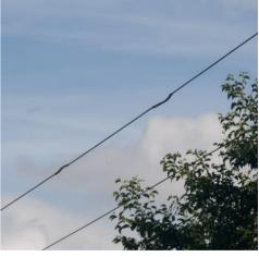
Twisted mid-span joints
