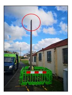
Chunk of failed concrete from lighting column caused the top extension arm to fall to ground
