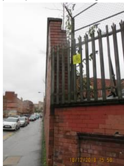
Top section leaning towards public footpath with vegetation growing through structure
