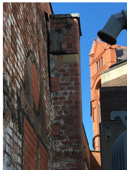
Paradise Street – wall and support pier separated and steel degraded
