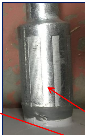
Figure 5. Correctly Compressed Henley Insulator
