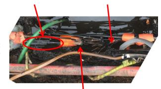
Flashover between L1 connector and inadequately covered neutral/earth wires
