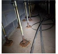
Where significant corrosion is found timber boards will be laid over the tiled floor as an interim measure to allow safe access and egress within the substations until the struts are replaced. This arrangement is now in place at Yarborough Road 132/33kV and also Santon 132/33kV substations along with signage.
