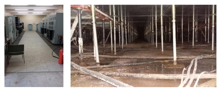
A recent 159 report identified significant corrosion to the lower section of some of these struts at Yarborough Road 132/33kV substation in Grimsby. As a result of these findings a programme has been created to identify all substations with this type of construction to allow a full condition survey to be carried out.
