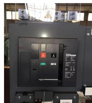
Figure 2: Schneider LV ACB
