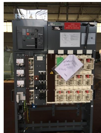
Figure 1: Schneider Shielded LV Board
