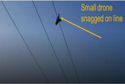
On the 27<sup>th</sup> June, 2019 at approximately 9pm, a member of the public came in contact with a 10kV 3 phase overhead line at Cabinteely public park, South County Dublin, while trying to retrieve a drone with a long scaffold pole. The drone had become entangled in an outer phase, mid span on the line. The individual appears to have received an electric shock and burns on his feet.
