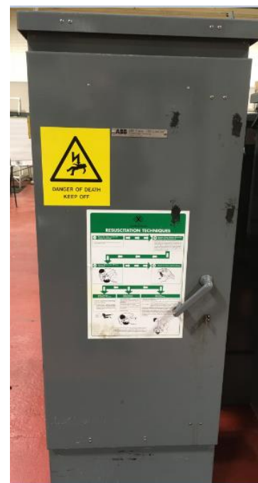
ABB Nitran Fully Shielded LV Fuse Cabinet – Transformer Disconnecter
