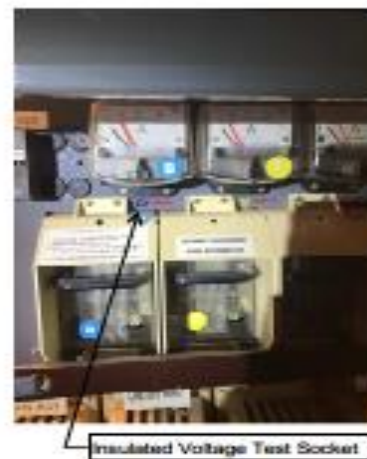
Fuse Cabinet door opened – Transformer Disconnecter Test Sockets
