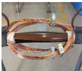
Prepared Joint prior to shrouding being applied
