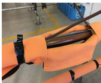
Shrouding applied to exposed metalwork
