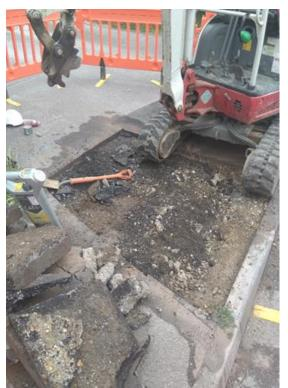
A Contract Partner was excavating an area of footpath to allow a new connection to take place. Following good practice, the Contract Partner used plans and CAT scans to locate the presence of buried cables before using a dust suppressed floor saw to cut the tarmac to be removed.
