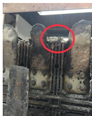
Fig 2: Suspected location of short circuit caused by bolt
