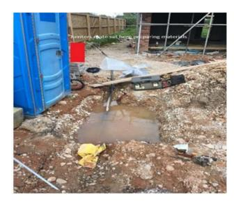
The IP had his back to the scaffolding and was overlooking the joint bay, preparing materials for the task when the incident happened. Both the excavation (the joint bay) and where the IP was working, was approx.4.5 metres away from the scaffold, and although a START risk assessment had been carried out, the team did not acknowledge the scaffold or the upright board as a significant risk. The IP was taken to hospital where he was diagnosed as receiving a muscular trauma.
