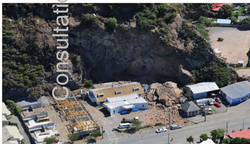
Figure 26: Substation Damage from Bolder - Wakefield Avenue
