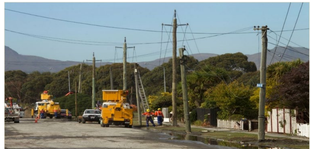
Figure 35: Emergency 66kV Overhead Line
