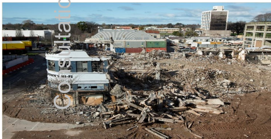
Figure: 30: Orion Office Demolition
