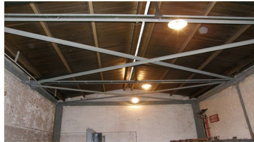
Figure 33: Substation Strengthening - Steel Framing
