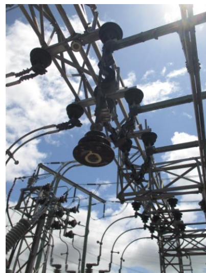
Photo showing the Pantograph section hanging prior to removal
