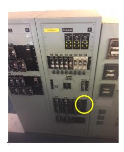
Whilst preparing for the Whirinaki (WHI) Substation Management System (SMS) project, one of the steps prior to work commencing was to check/confirm the position of all the switches on protection panels D2 and D3.
