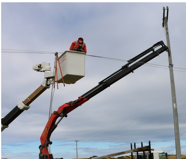
Conductor supported on the bucket
