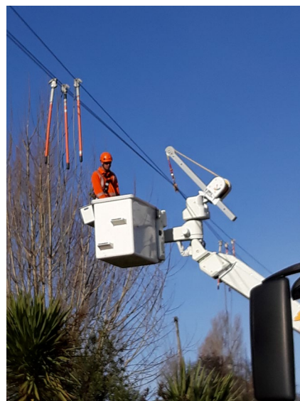
Conductor supported by the winch
