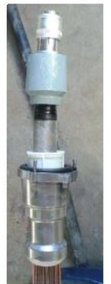
Photo #3 – Compression cone and insulating part installed
