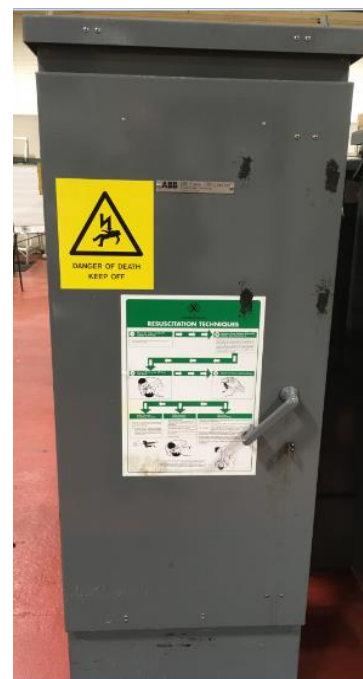
ABB Nitran Fully Shielded LV Fuse Cabinet – Transformer Disconnector
