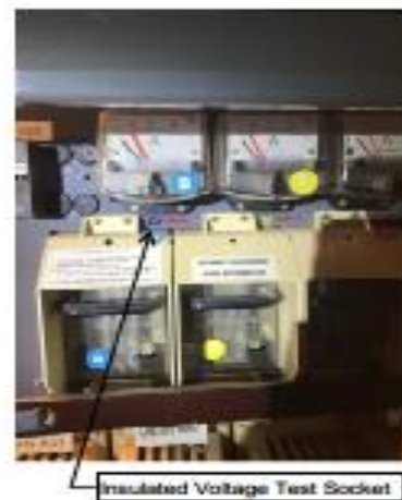
Fuse Cabinet door opened – Transformer Disconnector Test Sockets
