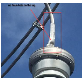
Figure 2. Example of lug with no 3mm hole
