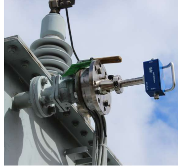
Figure 12. UHF antenna installed in oil drain valve
