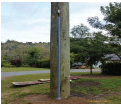
Pole down earth copper alternative
