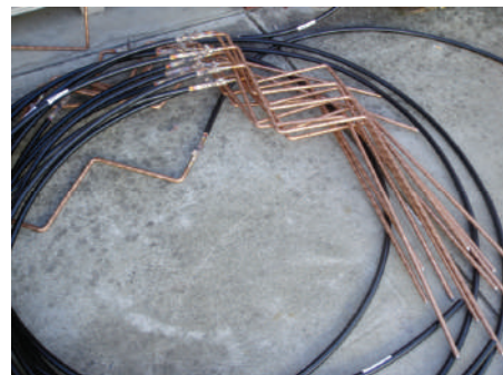
Substation Earthing tails –Theft deterrent
