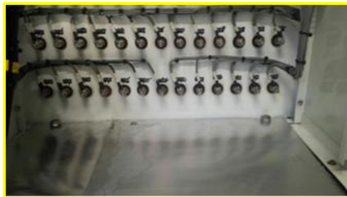
Test terminals & proximity to metal plate
